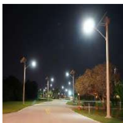
Solar Street Light
